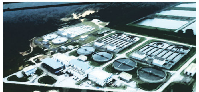
Regional Sewage Treatment Plant Kuala Sawah
