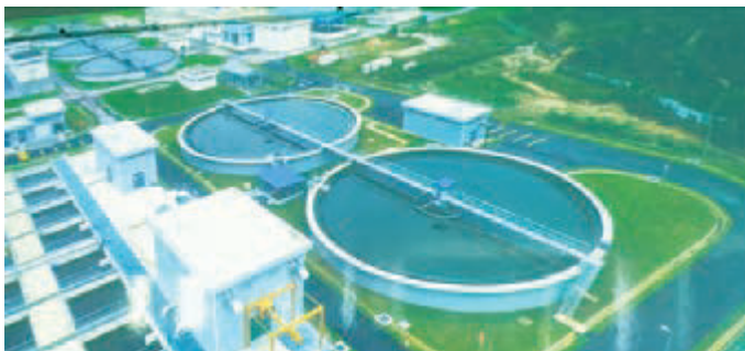
Regional Sewage Treatment Plant Kuala Sawah
