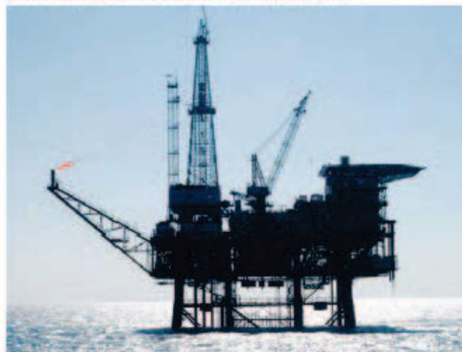
Figure 1: Fixed offshore platform (photo obtained from https://commons.wikimedia.org )
