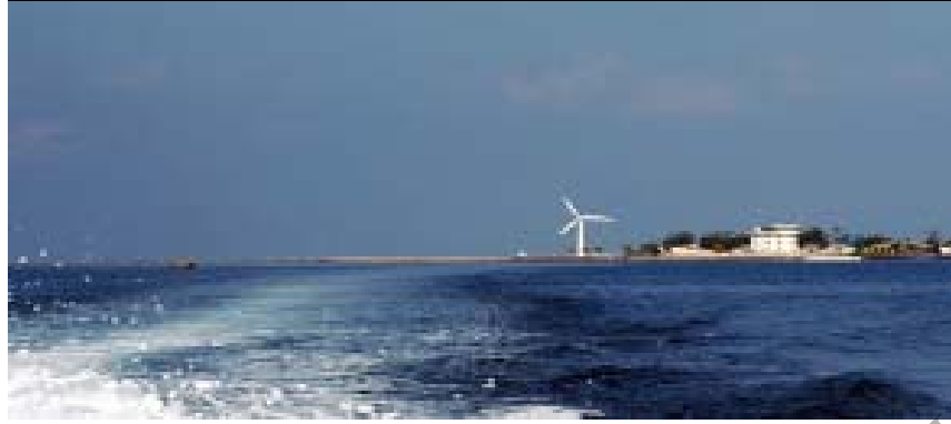
Figure : 150 kW wind turbine installed in Terumbu Layang-Layang, Malaysia.
