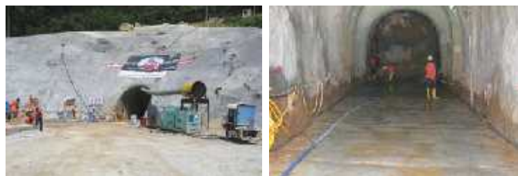
Tunnel construction within Lemoi river catchment
