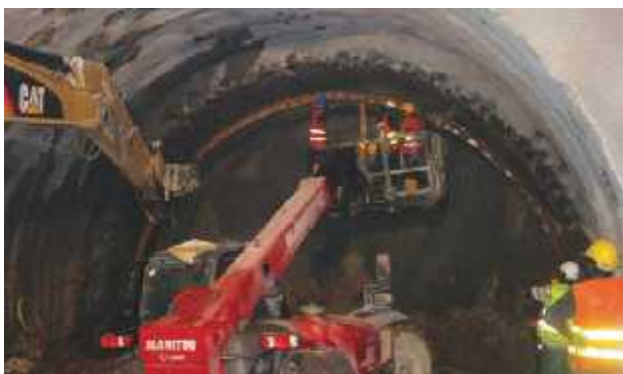
Construction of the Main Access Tunnel (MAT)
