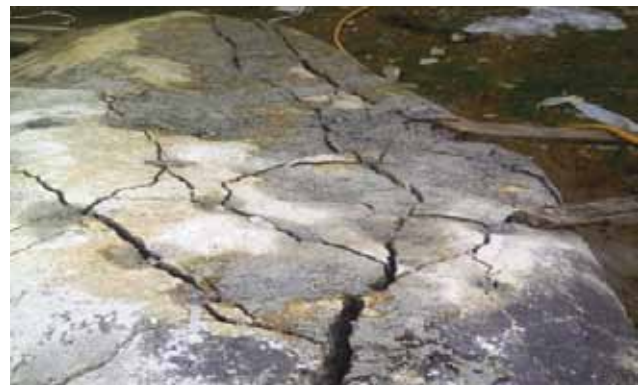
The boulders broken into small pieces using expansive cement
