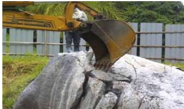
An excavator removing a broken rock outcrop
