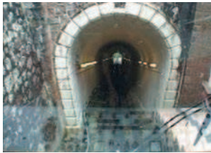
Figure 11: The same tunnel, reinforced to last
