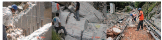
Figure 7: Using manual and hand-operated tools to break up rocks
