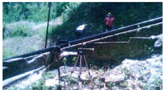
Figure 8: Noise monitoring during construction
