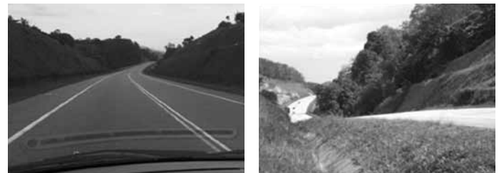
Figure 2: The case study area at Perak two-lane rural highway, horizontal and vertical curves
