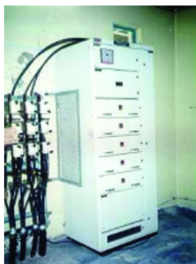
Figure 5: A low voltage capacitor bank at the distribution panel (2)
