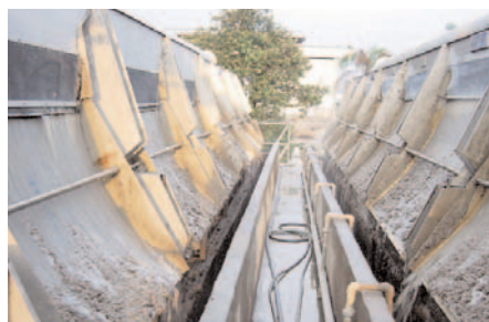
Figure 2 : Static screen
