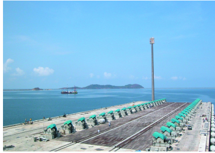
Figure 4: Illustrates the shiplift nearing completion
