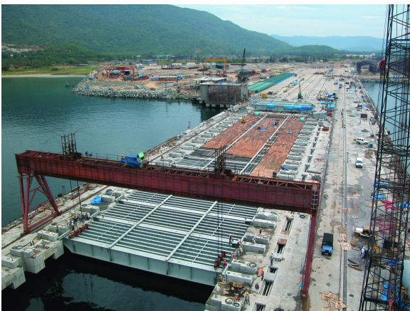
Figure 3: Platform erection gantry
