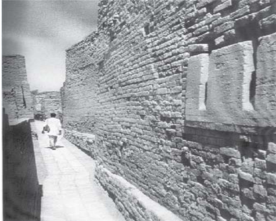
Figure 2.1. Mohenjo-Daro and Harappa built in 3000 B.C. (Lightweight Aggregate Concrete : Science, Technology and Applications, Chandra, S., and Bertsson, L.)
