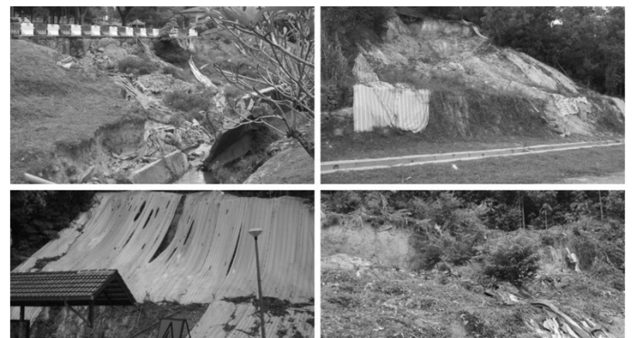
Figure 2: Landslides occurred in UKM Bangi Campus
