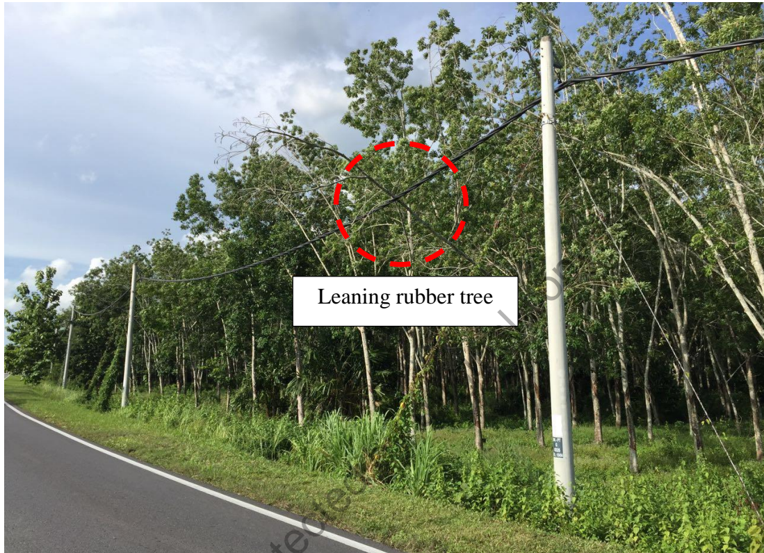
Figure 1.2: Leaning rubber tree on the 33 kV overhead power cables at Felda Chuping, Perlis, Malaysia.
