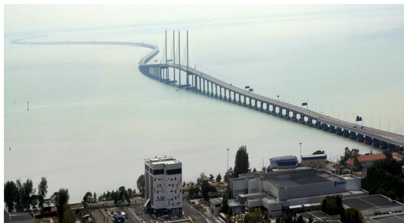
Figure 1. Overall view of Penang second bridge.
