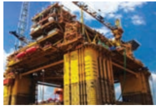
Gumusut-Kakap Semi-Submersible Floating Production System (FPS)
