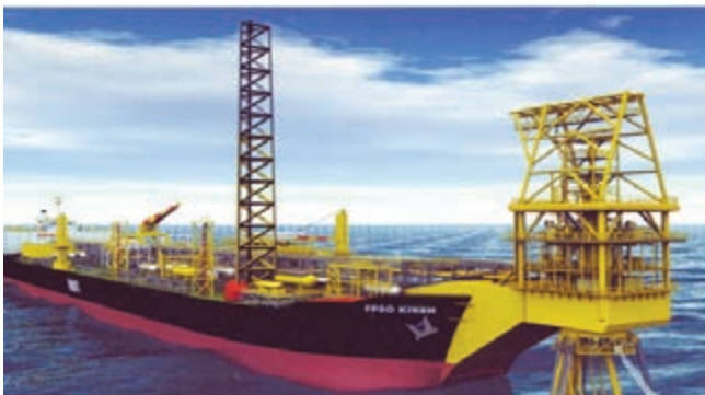
Figure 3a: External turret with the mooring lines and risers [Reference 4]
