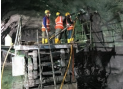
Figure 6: Rock dowel installation
