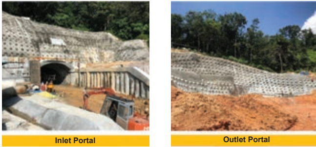
Figure 9: View of portals
