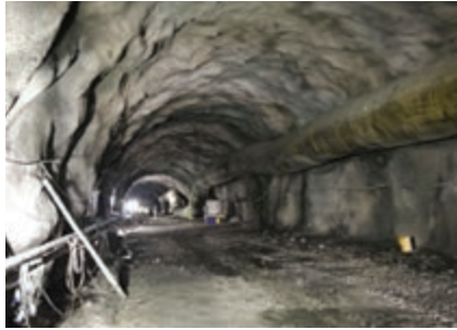
Figure 7: Fibre reinforced shotcrete lined rock face
