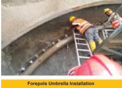
Figure 5b: Typical tunnel support
