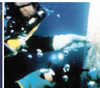
Figure 6: Level 3 inspection on a steel pile using ultrasonic devices [7]
