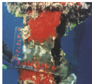
Figure 5: Level 2 inspection on a steel pile [7]
