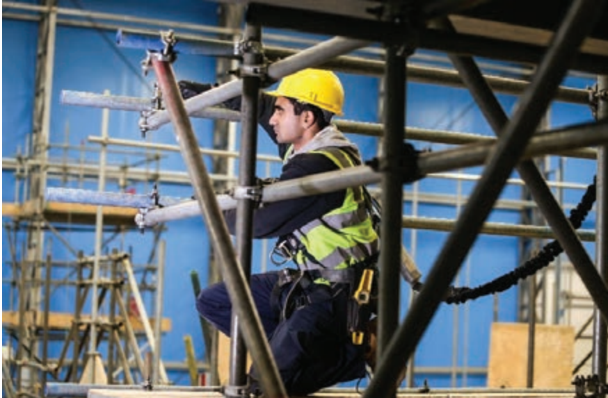
HuC scaffolding work on topside facilities
