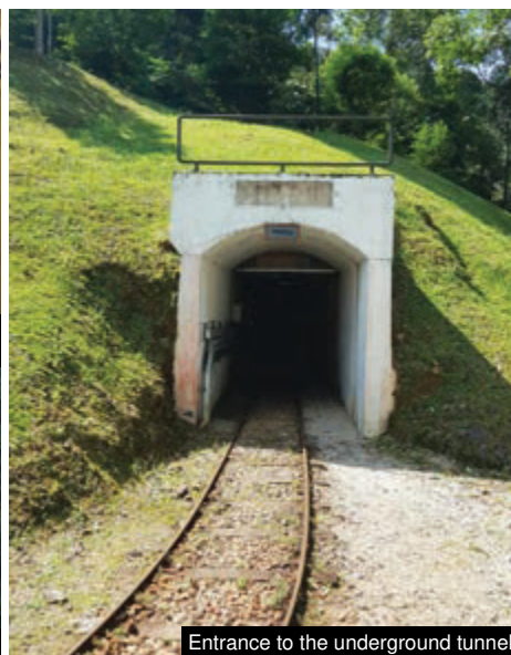
Entrance to the underground tunnel
