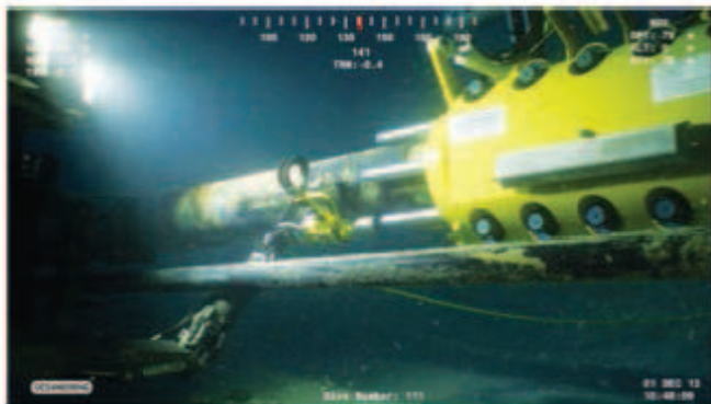
Subsea repair clamp installed by ROV
