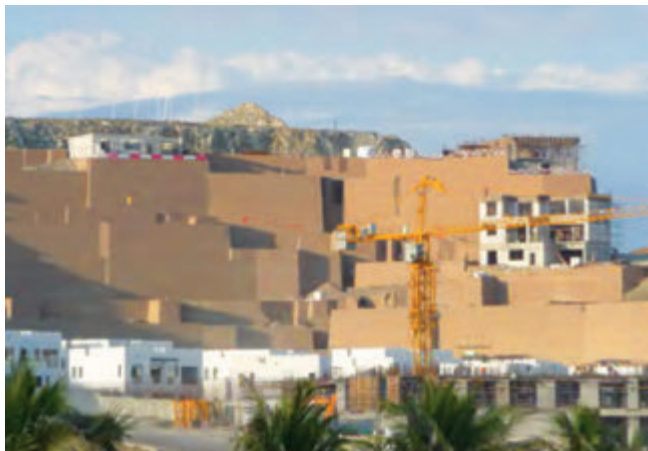
Figure 1: Example of Reinforced Soil Structures
