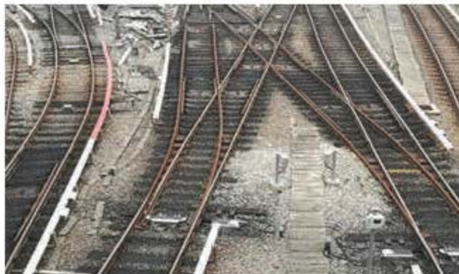
Modification of Existing Diamond Crossing
