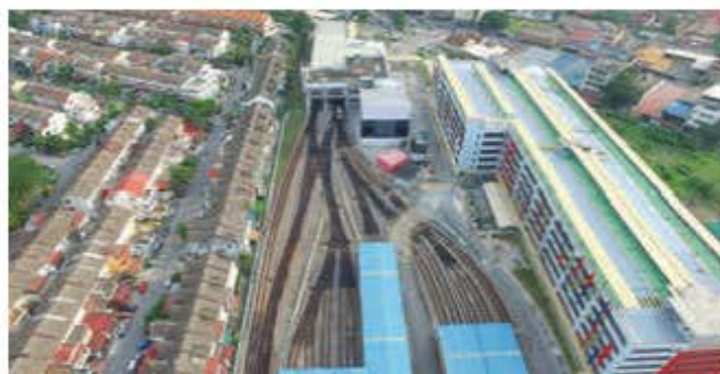
Northern view of Ampang Depot
