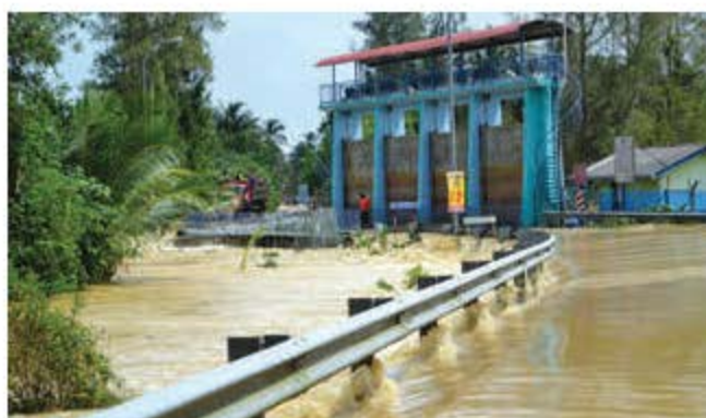
JPS uses Selehong Watergate to control water flow during floods in Tumpat, Kelantan.
