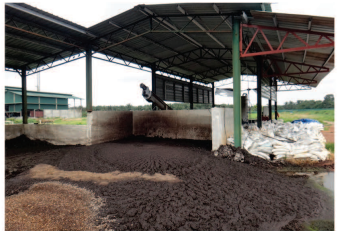
Photo 4: Solid storage bunker
