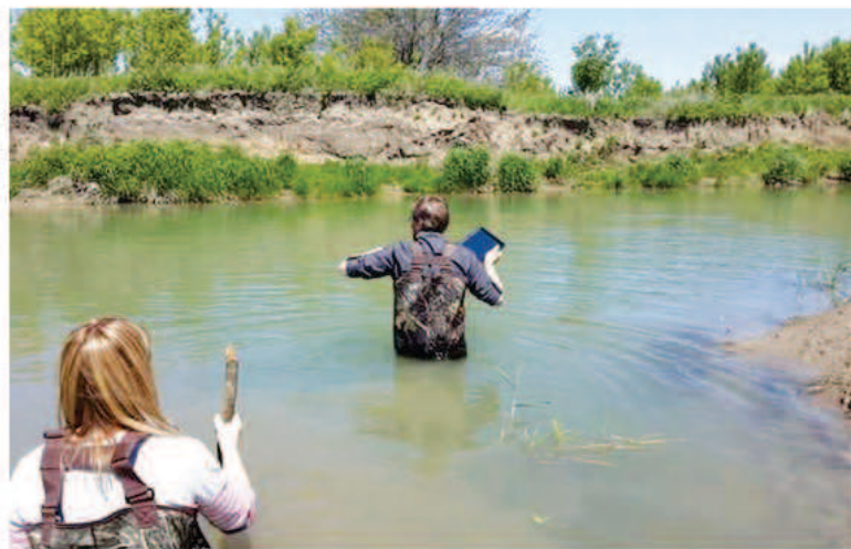
River Assessment and construction site inspection on water quality violation with Water Quality Inspector
