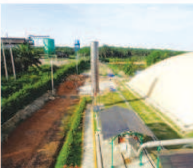
BIOGAS PROJECT-METHANE GAS CAPTURING
