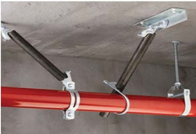
Lateral and longitudinal sprinkler pipe seismic bracing (source: http:// www.naffcoflow.com )
