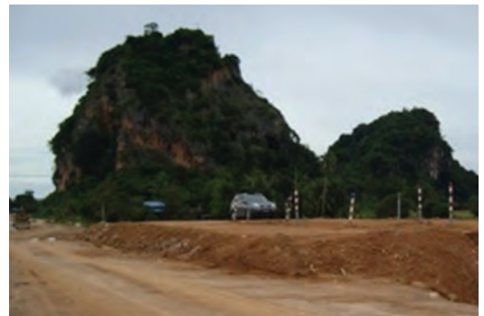
Photo 2: Photograph of completed test embankment
