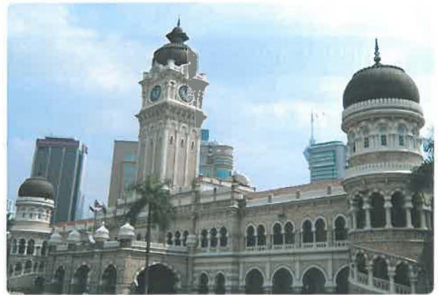
Figure 1: Non-Shabby Sultan Abdul Samad building (1897) using fired clay bricks as main construction materials.
