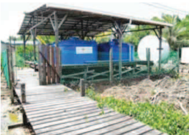
Completed rainwater harvesting system at Rumah Juing
