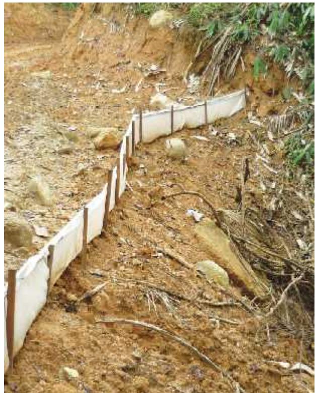
Figure 3: Provision of a silt fence on site
