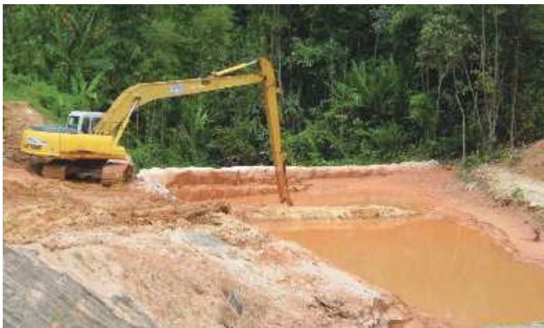
Figure 4: Removal of sediment from silt trap
