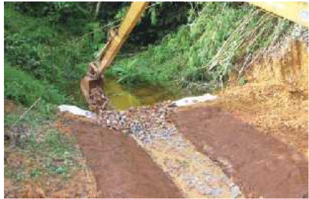
Figure 1: Construction of Check Dam
