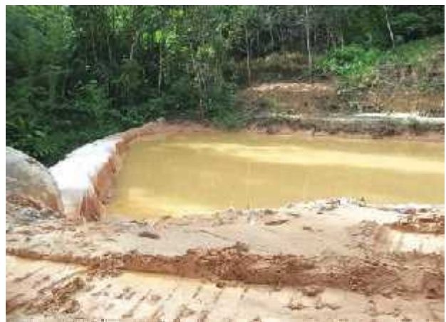
Figure 2: Silt trap on site
