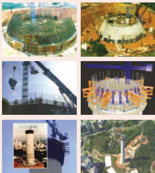
Engineering feat: The erection of KL Tower concrete shaft (Source: YTL)
