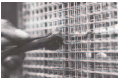
Figure 3: Reinforcing wires and mesh
