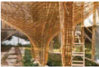
Figure 3: Reinforcing wires and mesh
