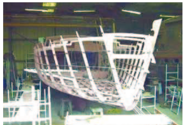
Figure 2: Steel frame for ferrocement hull construction
