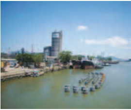
Photo 1: Completed piling work for pier
