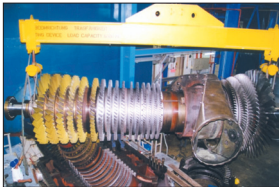
Gas turbine rotor being re-fitted to the machine after refurbishment
