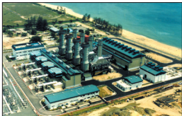
YTL's 808MW Combined Cycle Power Plant in Paika, Terengganu
