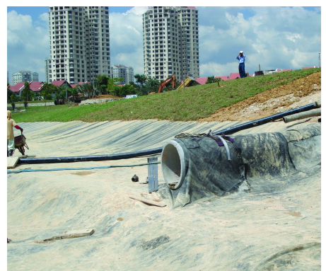
Figure 5: Liner termination at pipe penetrations
