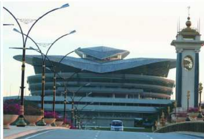
The Putrajaya International Convention Centre
