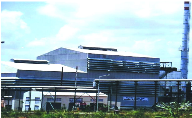
Courtesy: Sri Lakshmir Textile Ltd, Mysore, India. March 2001 Figure 3: Biomass Power Plant
