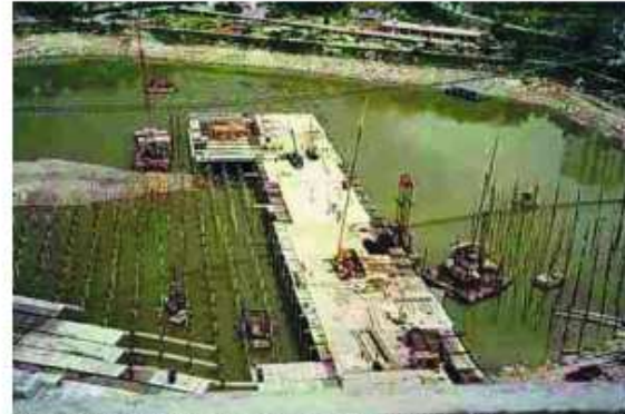
Figure 5: Aerial view the construction work in progress
