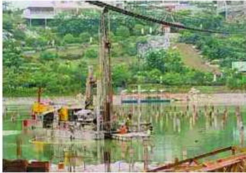
Figure 3: Installation of micropiles from a pontoon
