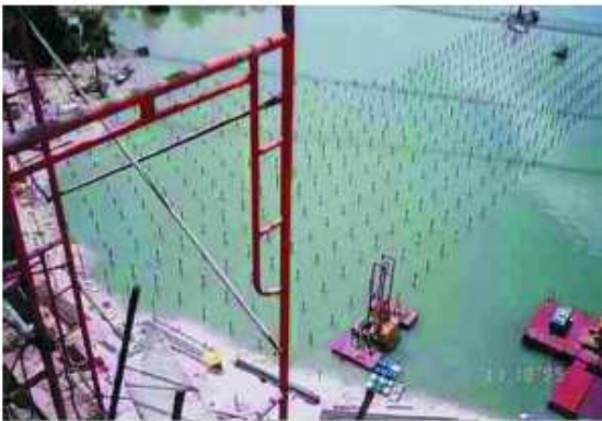
Figure 4: Aerial view of micropiling works
