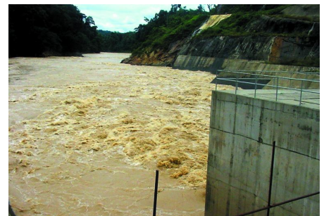
Figure 5: Downstream of the Cofferdam
