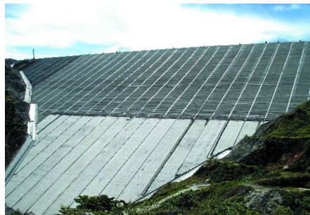
Figure 2: A view of the completed dam
