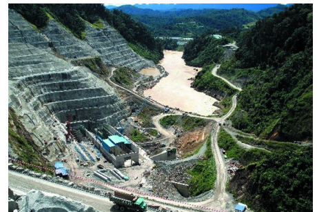
Figure 3: A view on how the dam has been gradually constructed
