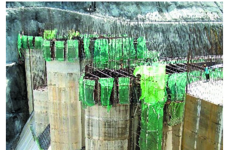
Figure 1: A side view on the construction of the huge Cofferdam which is still in progress
