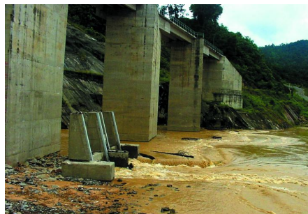
Figure 4: Upstream of the completed Cofferdam
