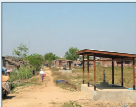
An ingenious collection system for rainwater, used where pond storage is not feasible. Water collects from the roof into a below ground tank and is hand pumped out when needed
