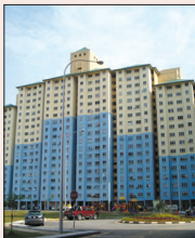
PPR Low Cost Flats at Taman Wahyu, Selayang, Selangor
