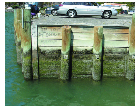
Figure6: Timber retaining wall used in marine conditions
