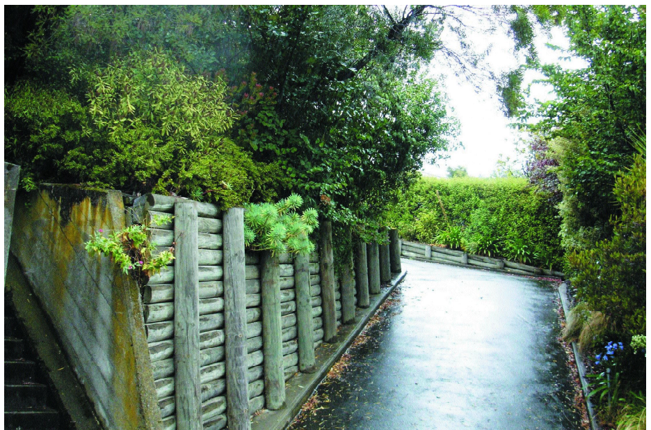
Figure2: Wood retaining wall blends with the landscape
