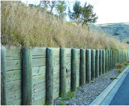
Figure3: Pole retaining wall
