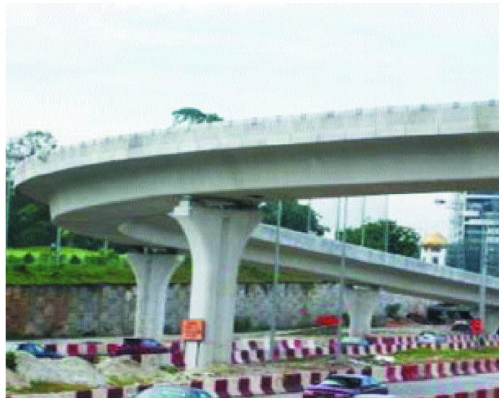
Figure 4: A completed prestressed concrete box girder ramp under Section 3
