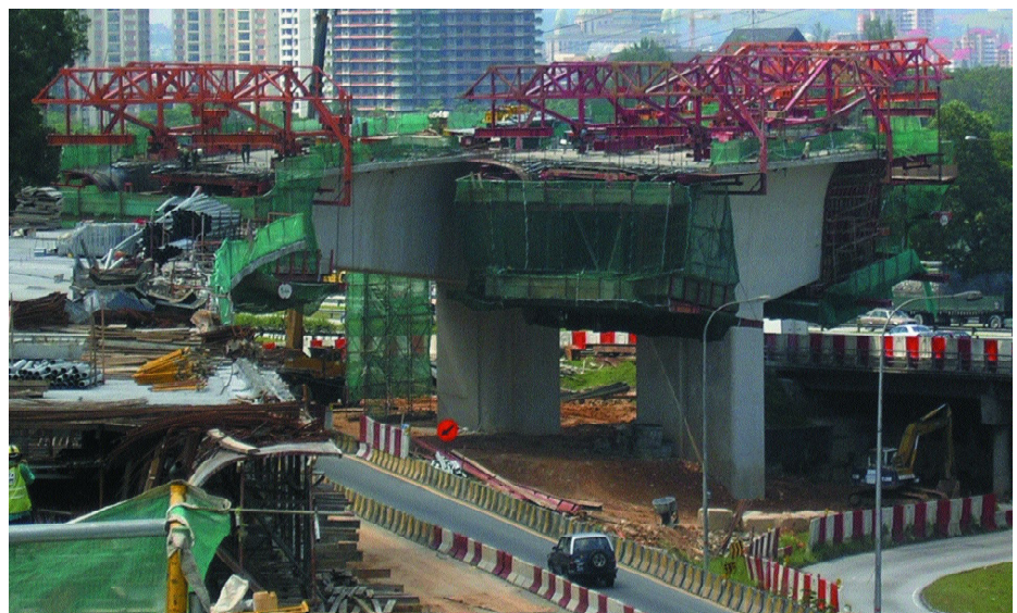
Figure 3: "Travelling" construction in progress at Section 2
