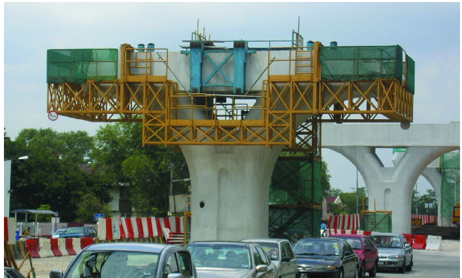
Figure 1: Y-shape pier at Section 1
