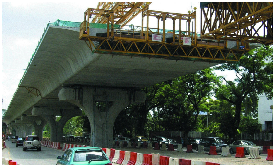
Figure 2: Precast concrete segmental construction at Section 1
