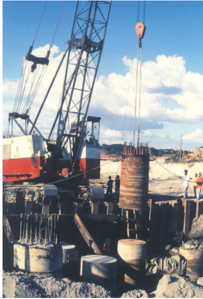
Figure 6: Dynamic pile test for a cast-in-place concrete pile
