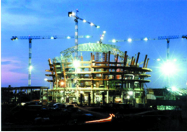
Putrajaya Convention Centre construction - Night View
