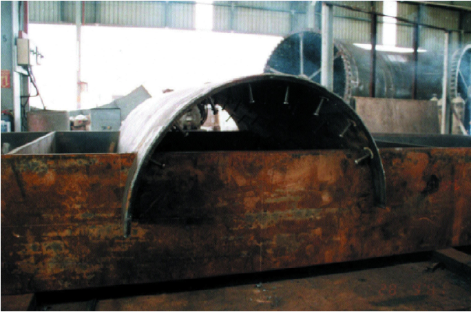
Figure 5: Plate Girder welded into half of Column Steel Node
