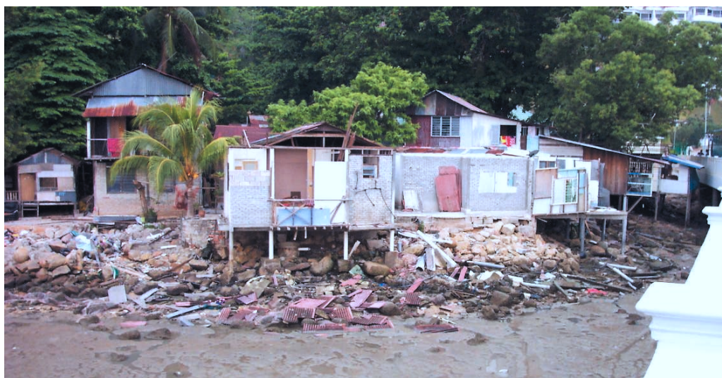
Photo 6: Severe damages from Tsunami Batu Feringghi
