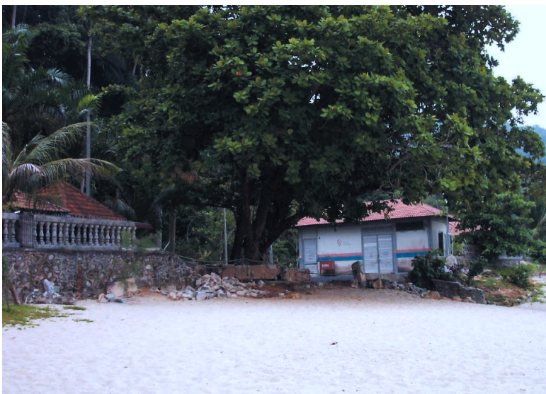
Photo 7: Damaged wall and loss of lives at Pasir Panjang beach
