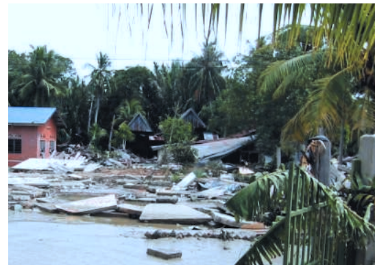
Photo 2a: Damage to houses at Kuala Muda
