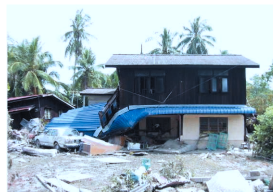
Photo 2c: Another view of damage to property at Kuala Muda
