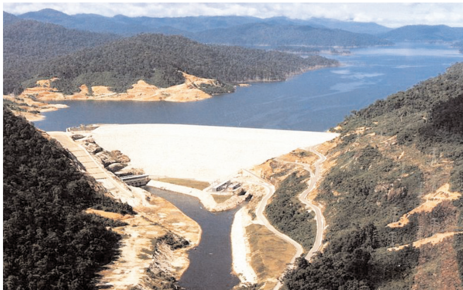
400MW Kenyir Hydropower Station in Terengganu
