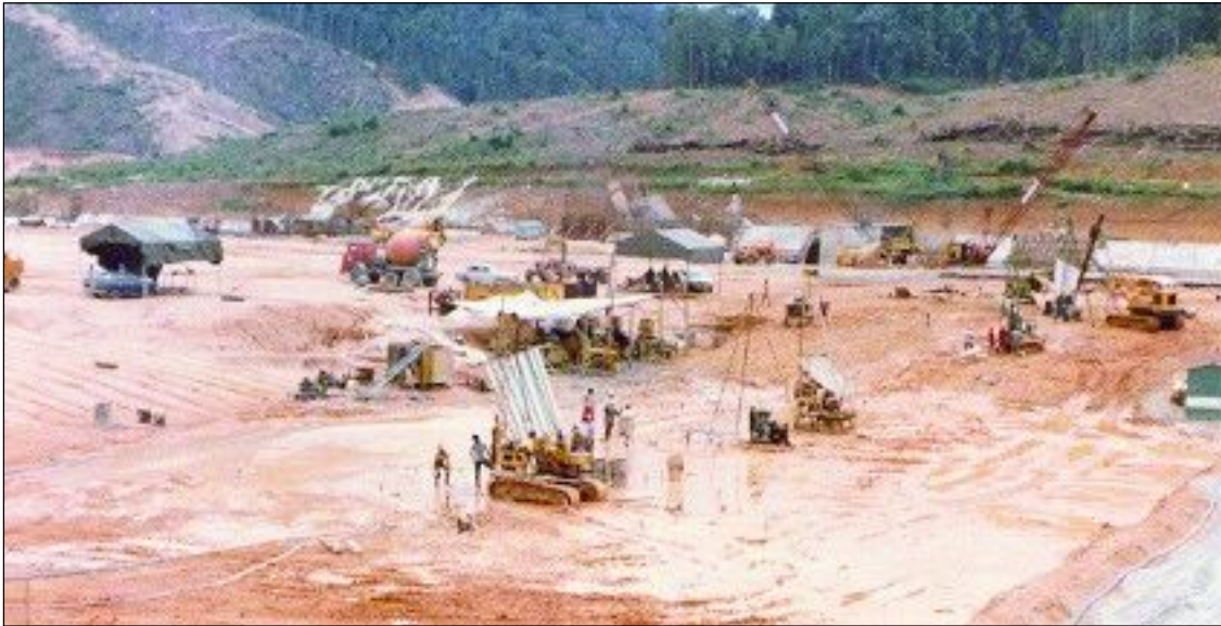
Figure 14: Foundation grouting at Batu Dam, K.L.
