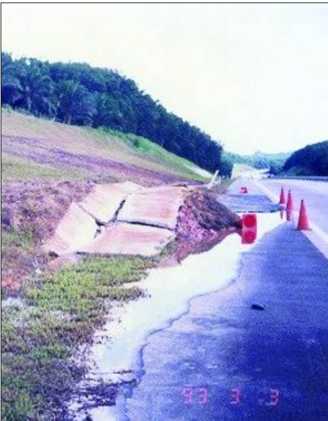
Figure 7: "Flattened" cut slope in graphitic schist, North-South Highway near Rawang
