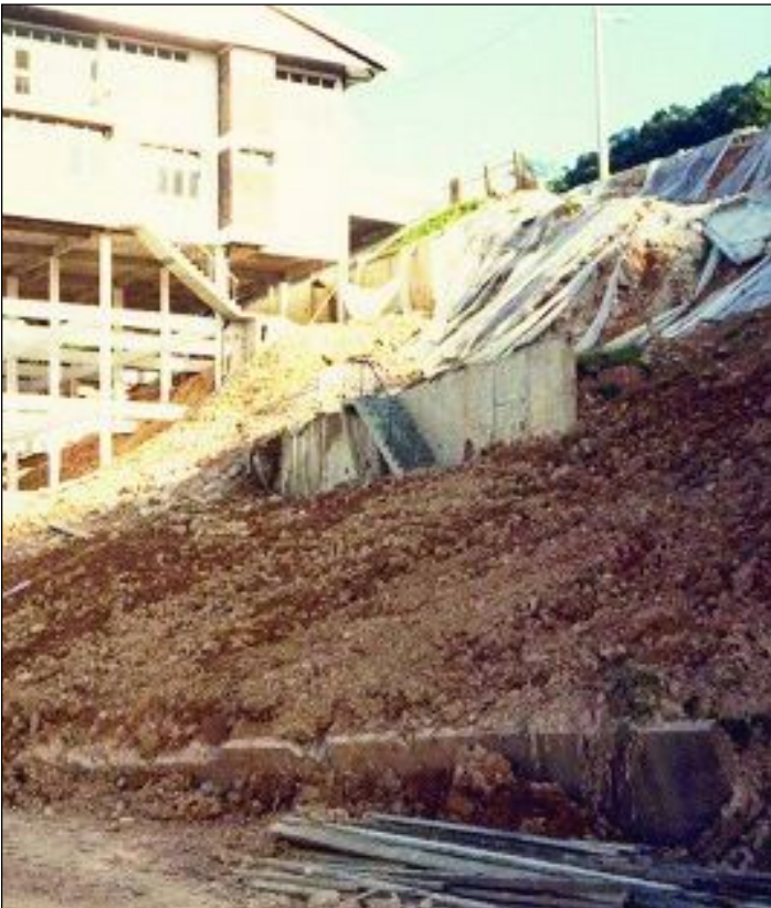
Figure 13c: Slope failures associated with housing projects in hilly terrains, Kuala Lumpur
