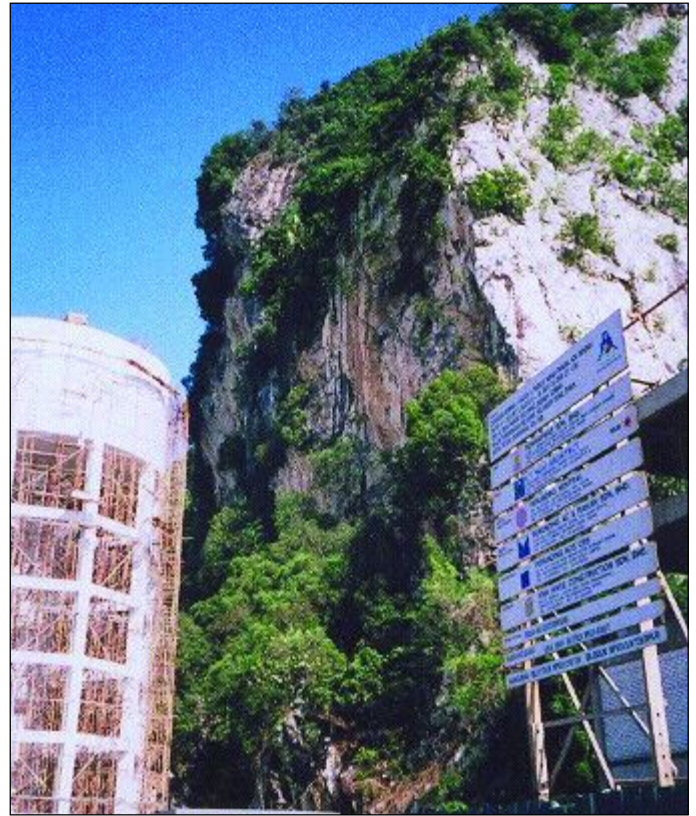
Figure 4: Water tank at Batu Caves limestone cliff, Kuala Lumpur
